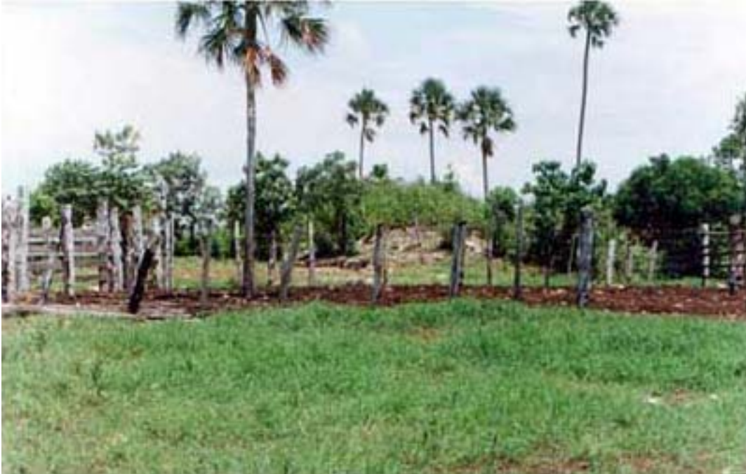
Photo 39. Structure at Site 11 located within the lands of a ranch.
