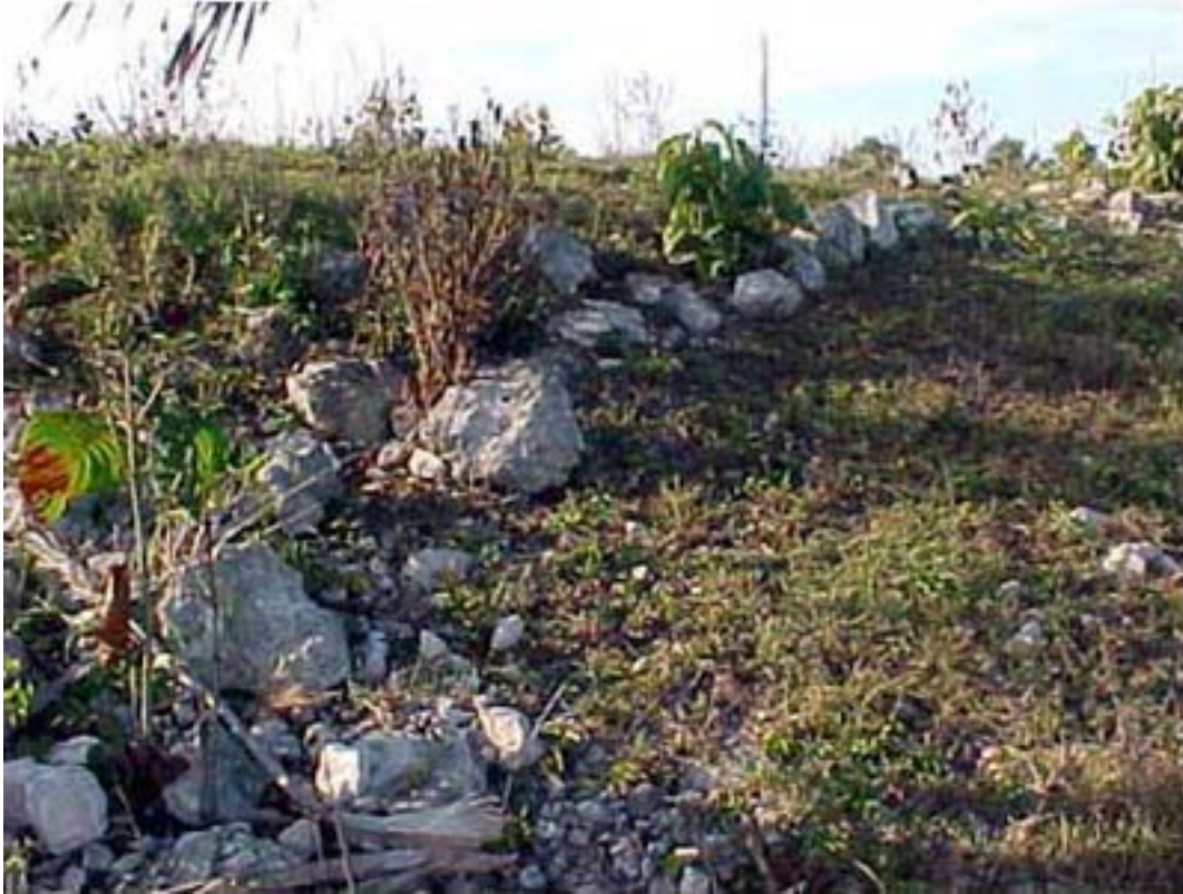
Photo 49. Retaining wall of a platform in Site 19, still visible.
