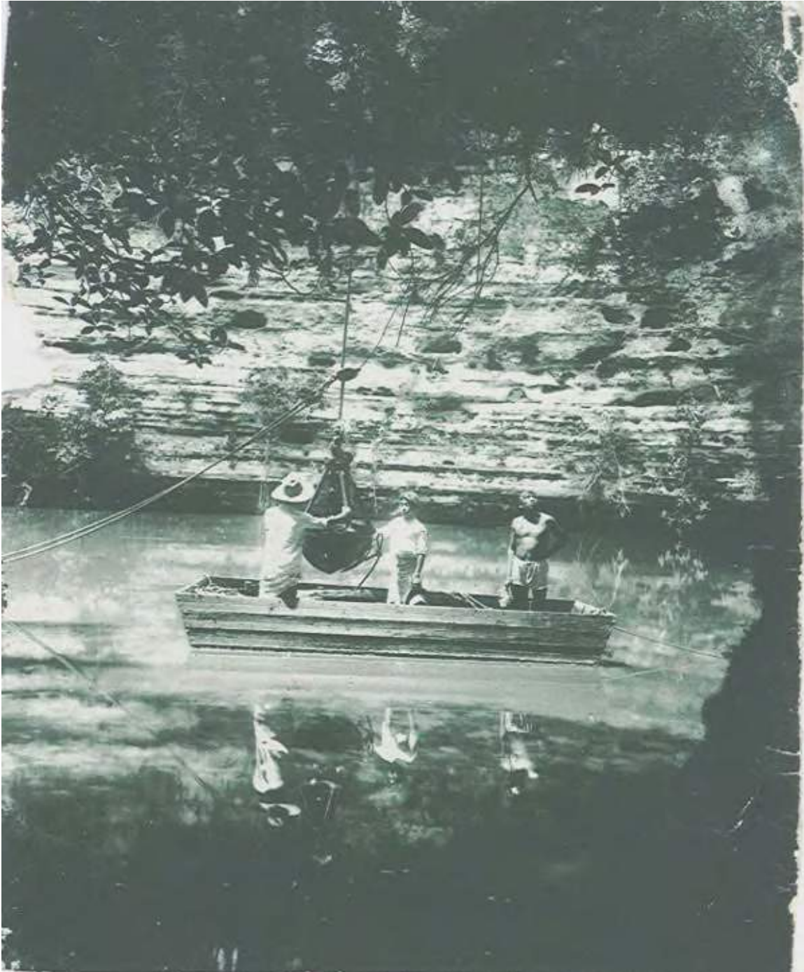
Figure 7. Placing the dredger on the raft.
