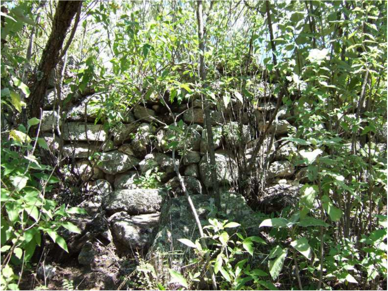
Figure 12: Stone Retaining Wall (Terrace C5 West)
