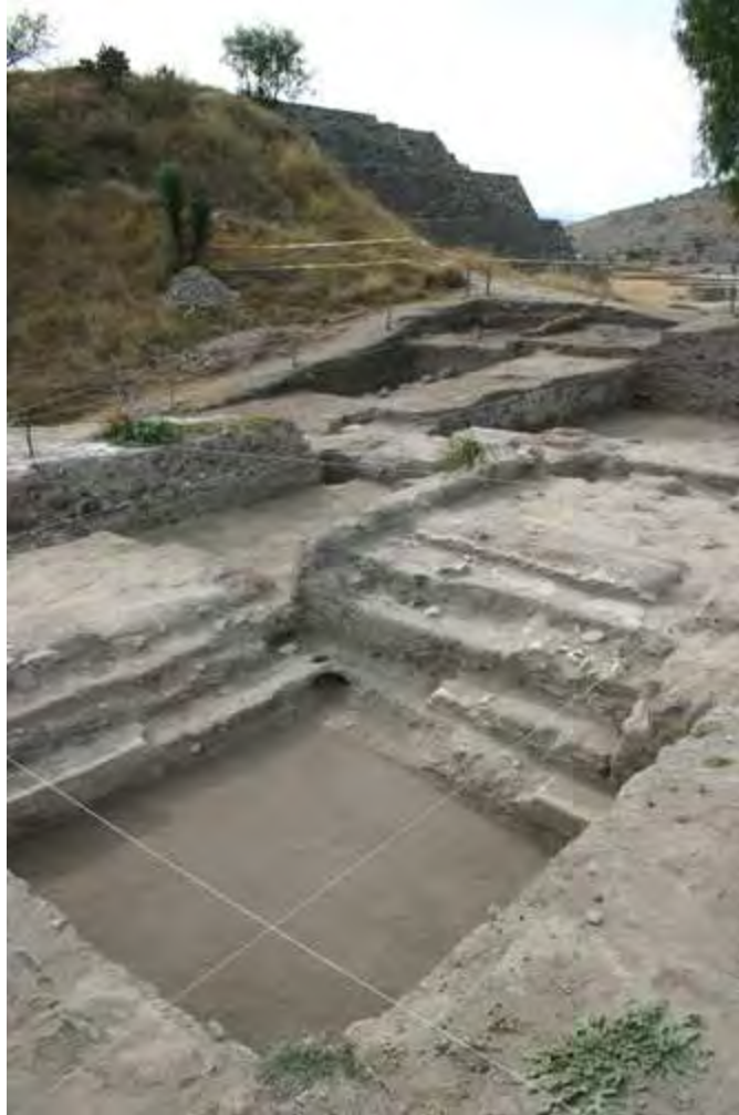
Figure 23. Tepetate slats were also used to build the stairways of the building (courtesy of Dan Healan).
