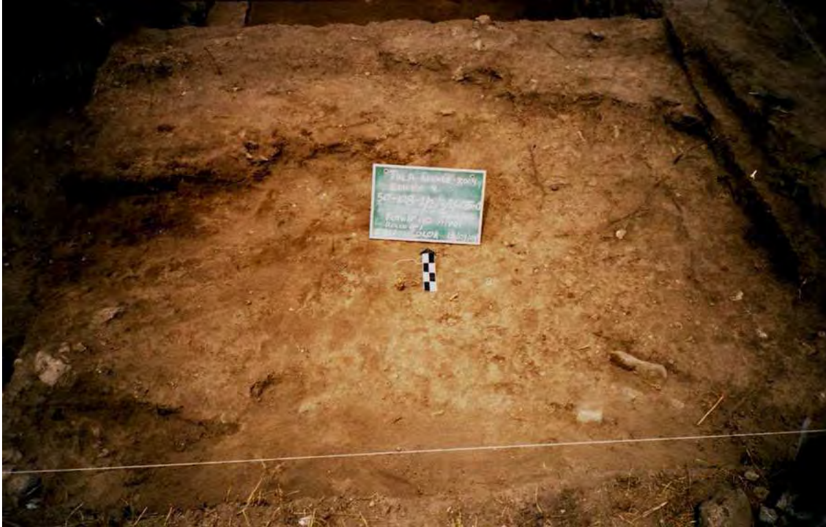
Figure 12. Detail of the adobe core as part of the building's foundations.
