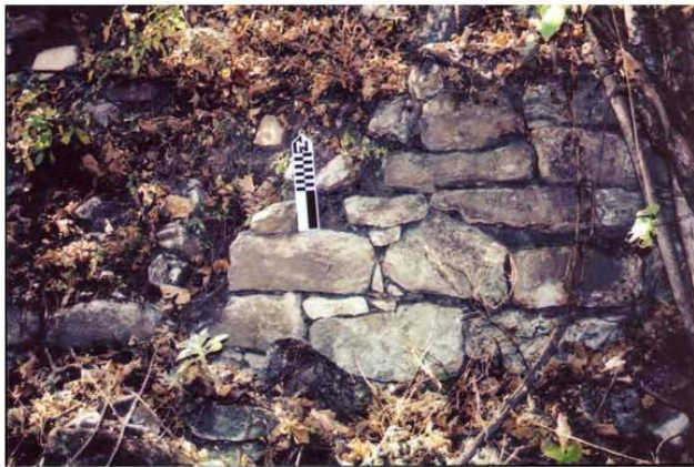
North Retaining Wall (Façade Partially Intact)
