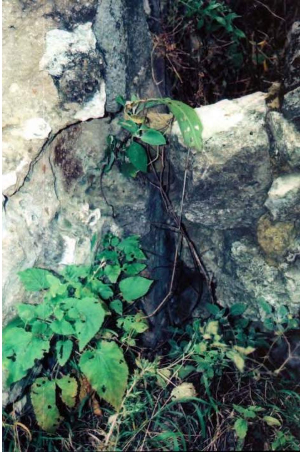
Figure 19. Structure 4 Wall Truncated by Church.
