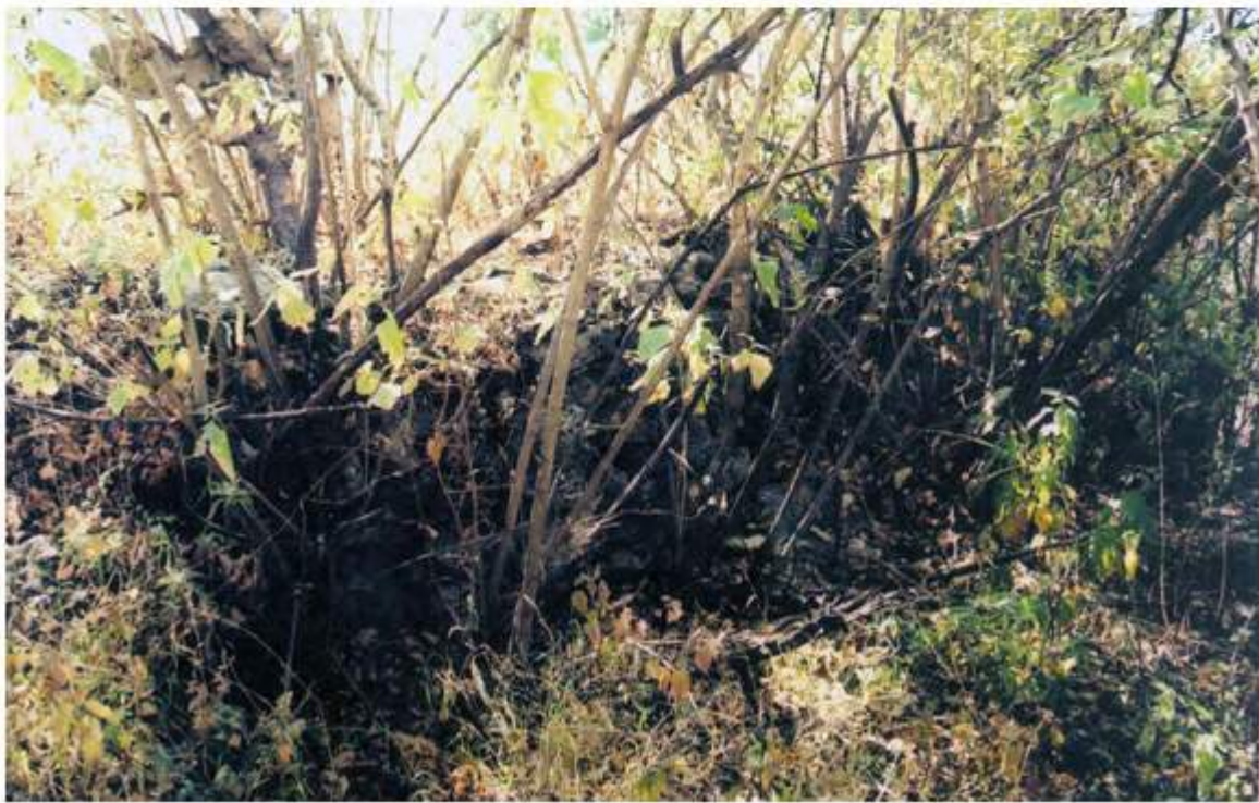
Figure 24. Platform 10 West Retaining Wall (Facing Stone).
