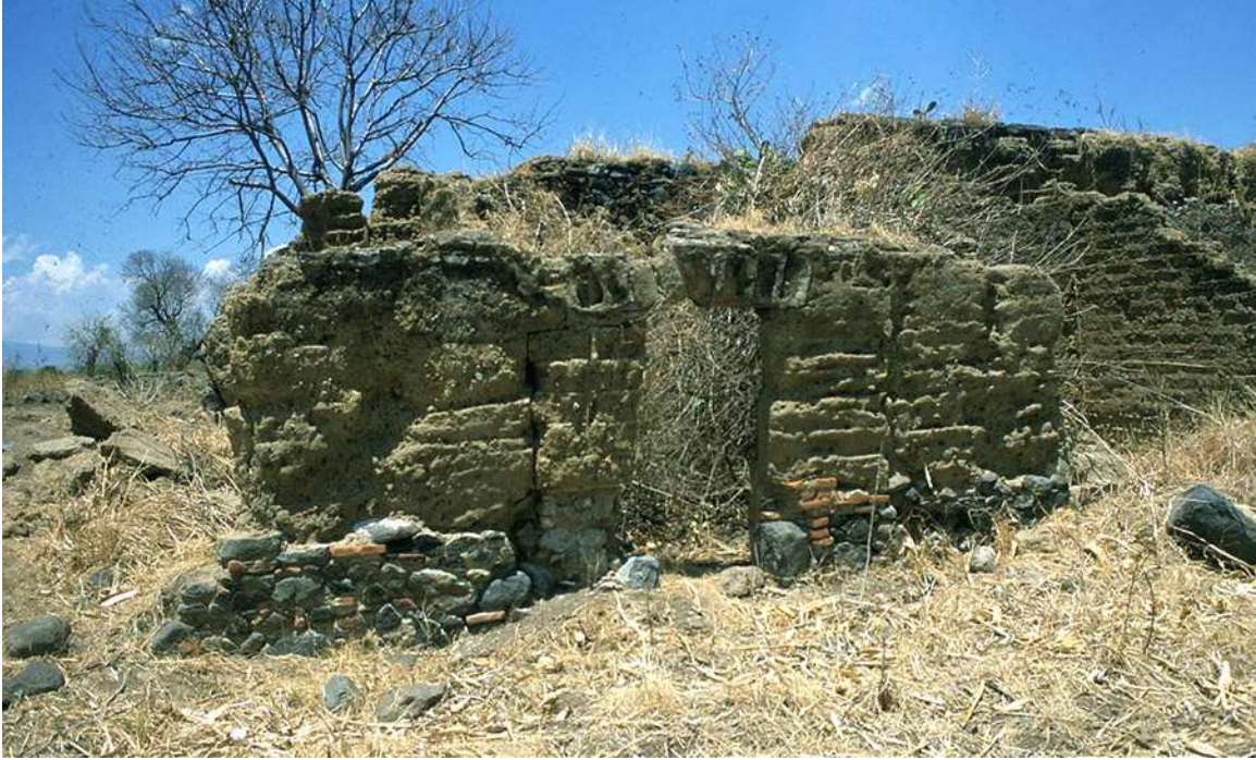
Photograph 3. Calpanería Room, well-preserved example.
