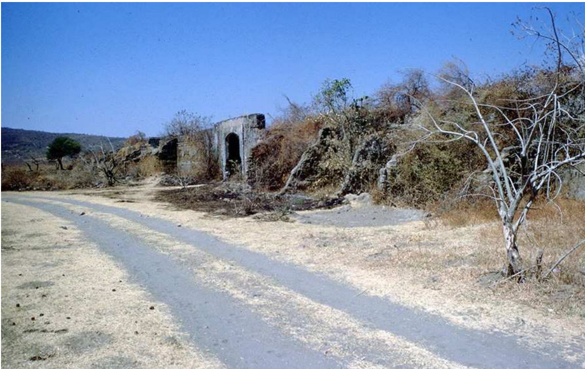
Photograph 1. Calpanería and Main Entrance.
