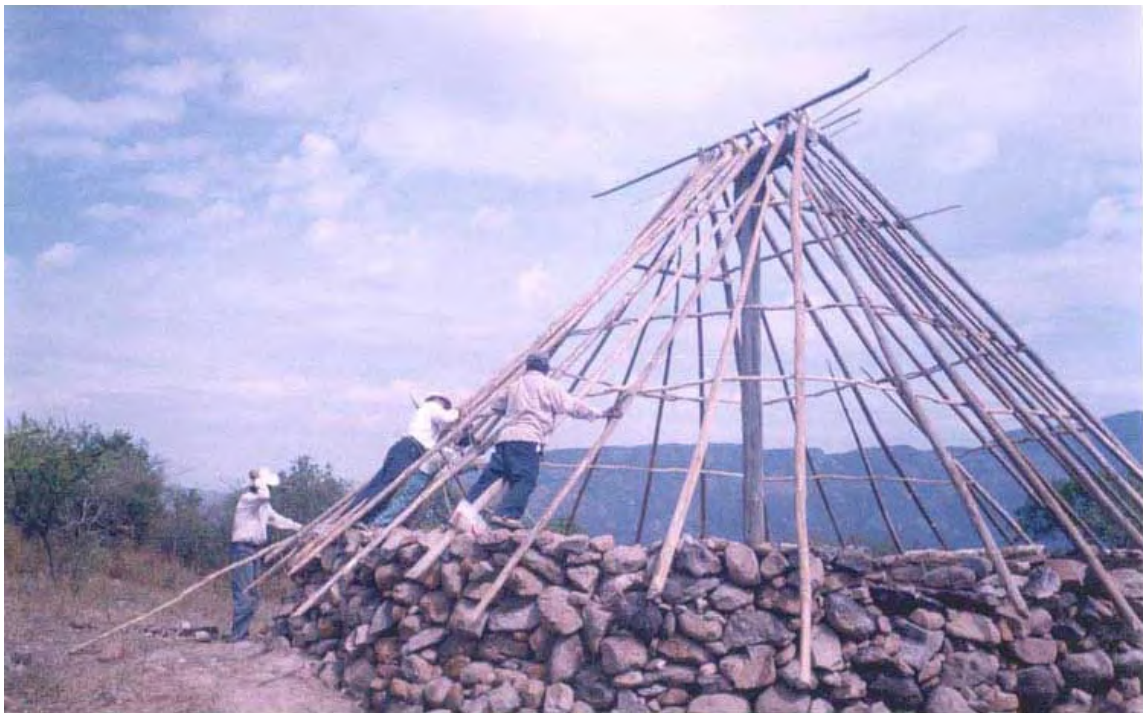
Figure 31. Temple's roof structure. Photo provided by Mr. Pablo Muñoz.
