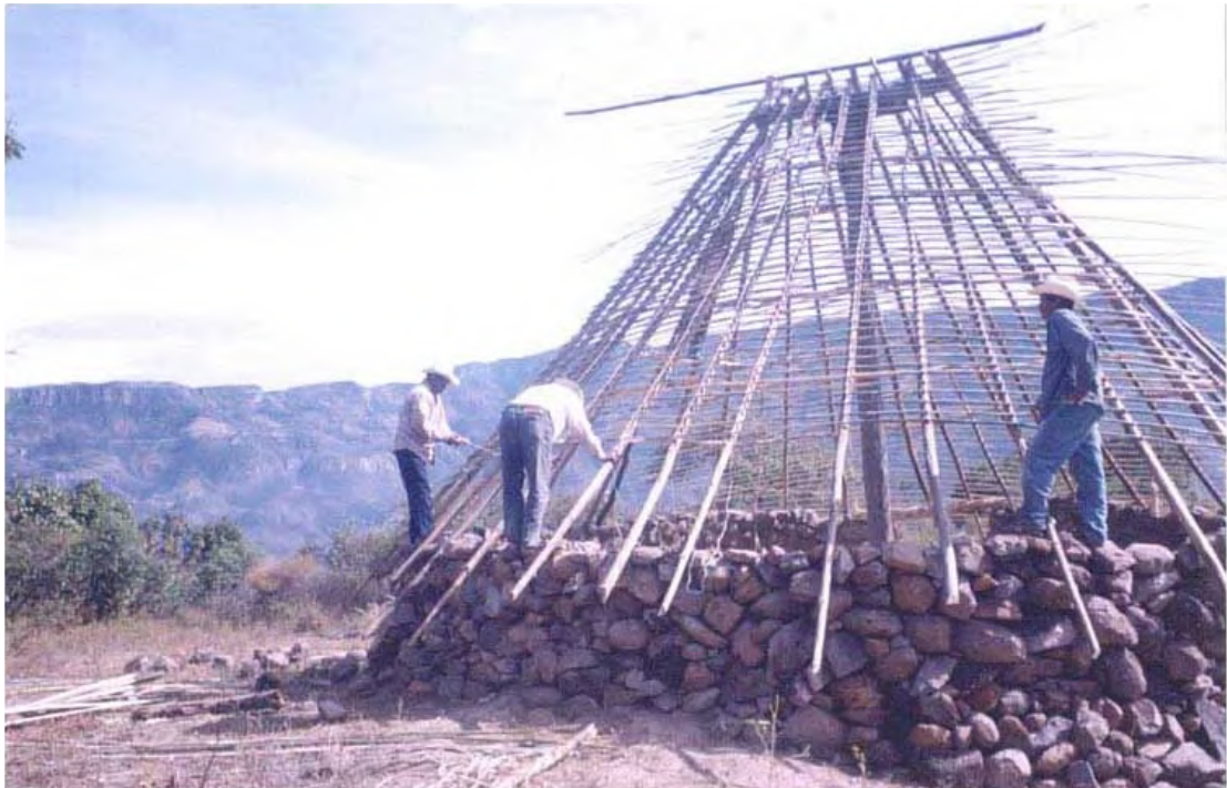
Figure 33. Temple's roof structure. Photo provided by Mr. Pablo Muñoz.
