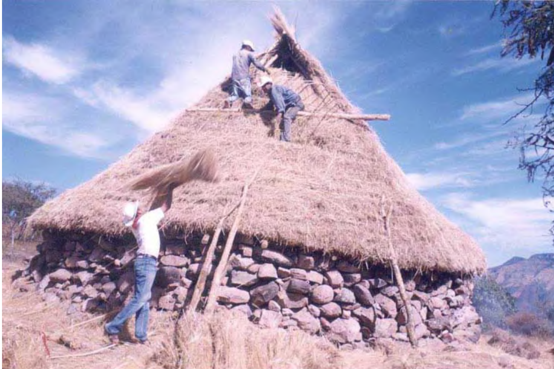
Figure 38. Building the Tuki's roof. Photo provided by Mr. Pablo Muñoz.
