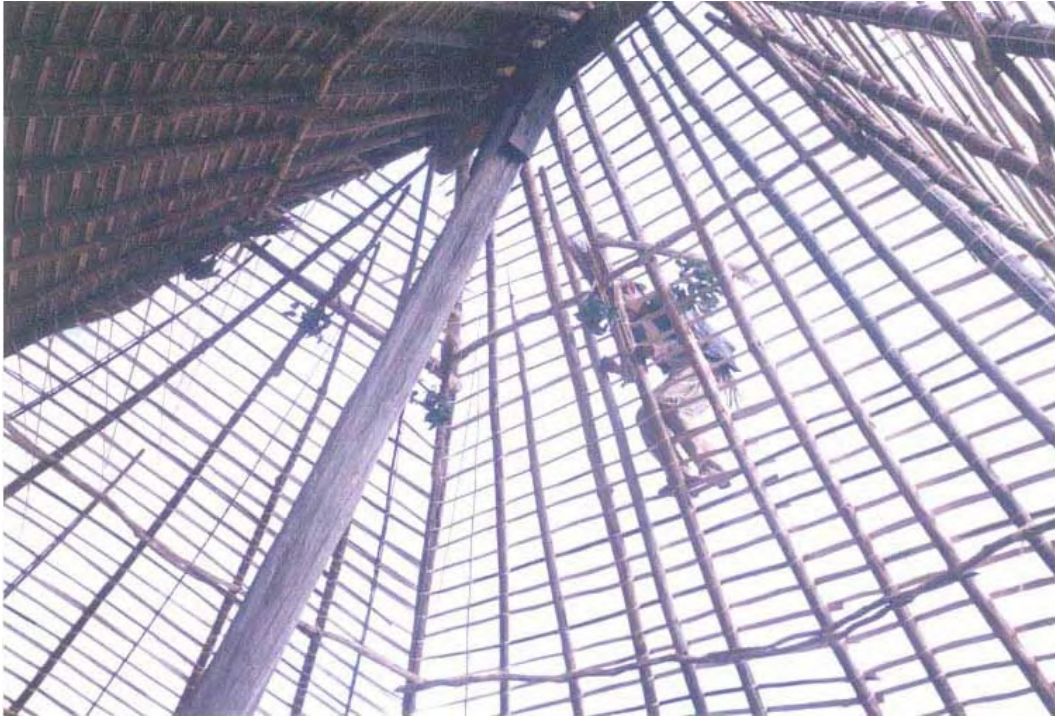
Figure 37. Building the Tuki's roof. Photo provided by Mr. Pablo Muñoz.
