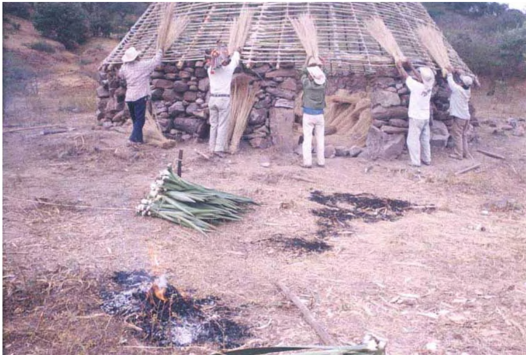
Figure 34. Building the Tuki's roof. Photo provided by Mr. Pablo Muñoz.
