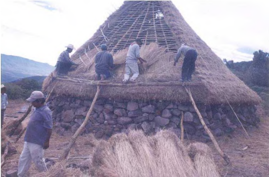
Figure 39. Building the Tuki's roof. Photo provided by Mr. Pablo Muñoz.
