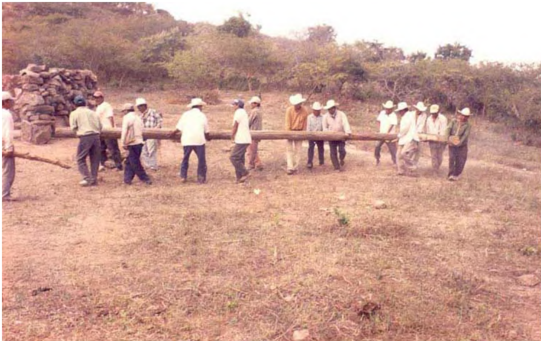
Figure 25. Putting the temple's central post in place. Photo provided by Mr. Pablo Muñoz.
