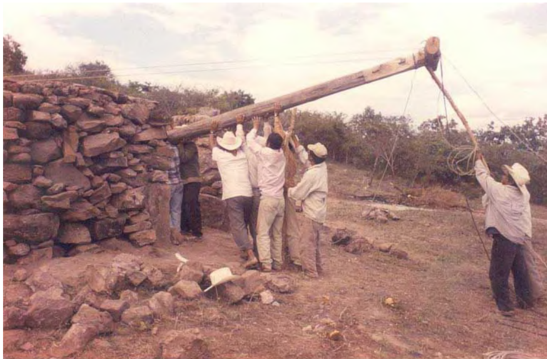
Figure 27. Putting the temple's central post in place. Photo provided by Mr. Pablo Muñoz.
