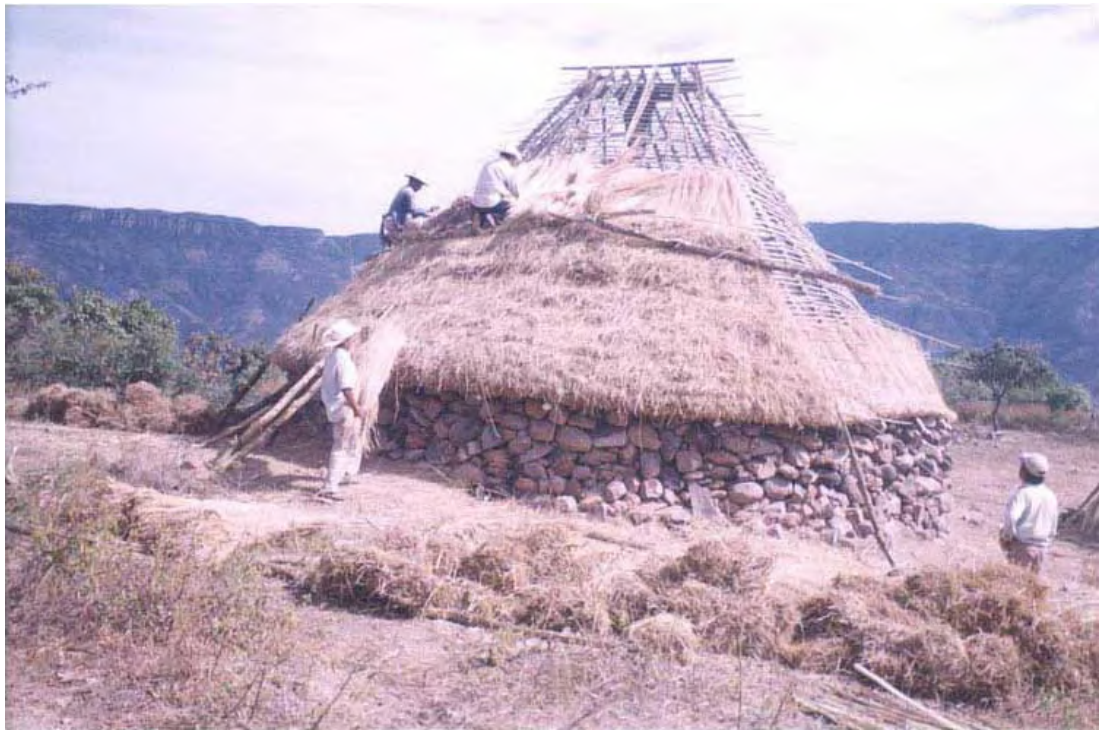
Figure 36. Building the Tuki's roof. Photo provided by Mr. Pablo Muñoz.
