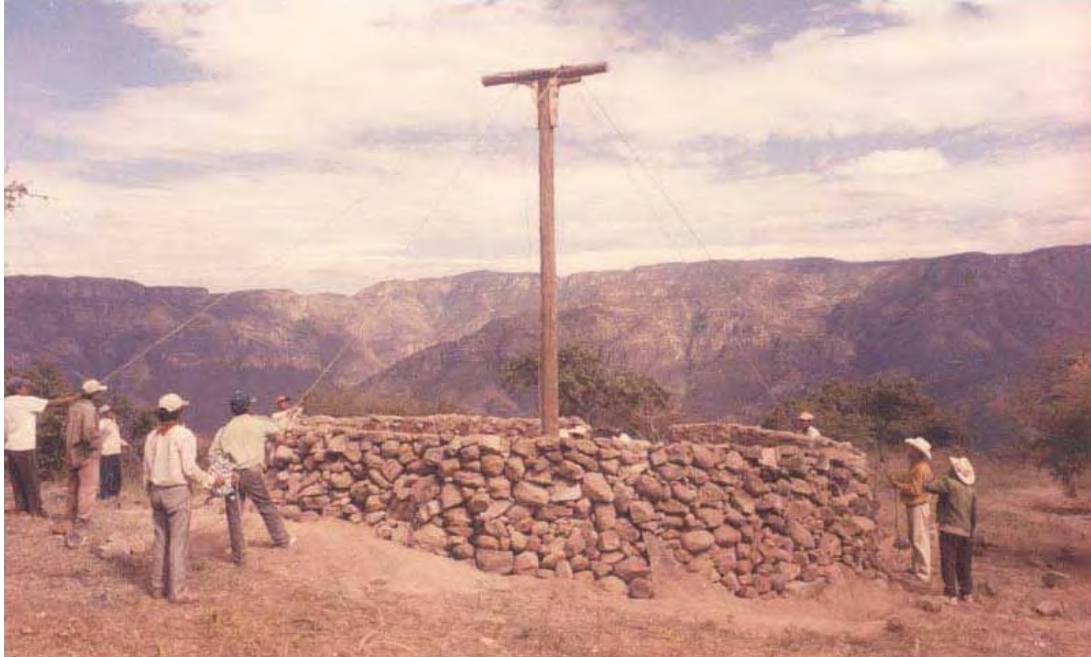
Figure 28. Putting the temple's central post in place. Photo provided by Mr. Pablo Muñoz.
