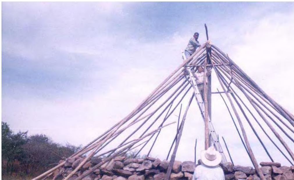
Figure 29. Temple's roof structure. Photo provided by Mr. Pablo Muñoz.
