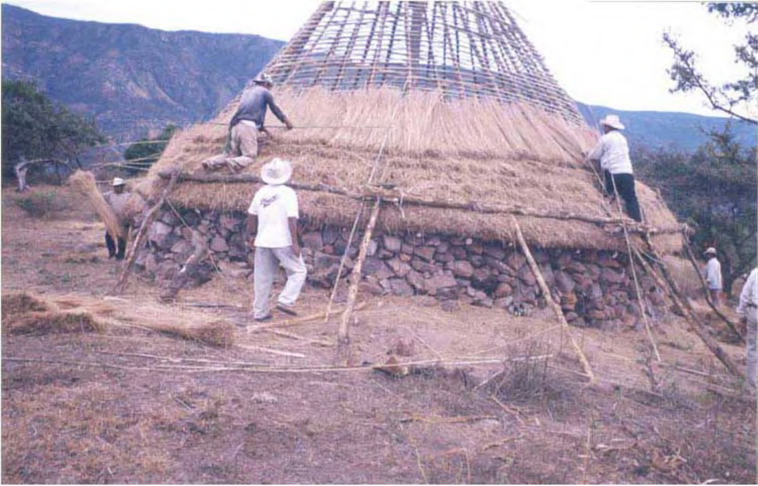
Figure 35. Building the Tuki's roof. Photo provided by Mr. Pablo Muñoz.
