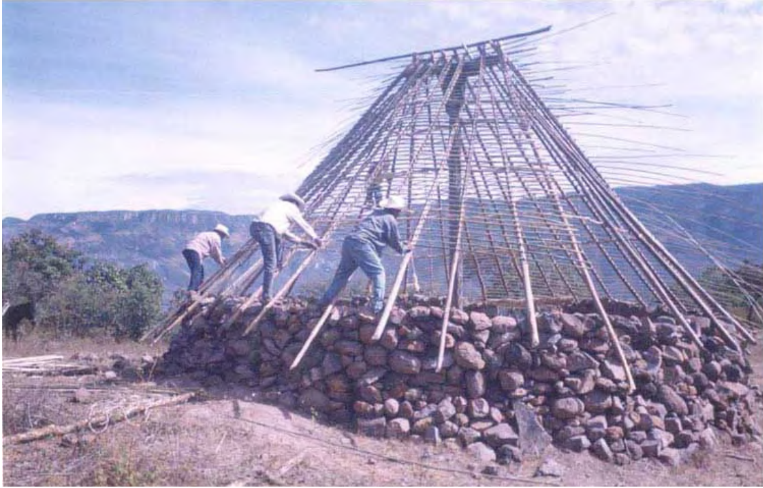
Figure 32. Temple's roof structure. Photo provided by Mr. Pablo Muñoz.
