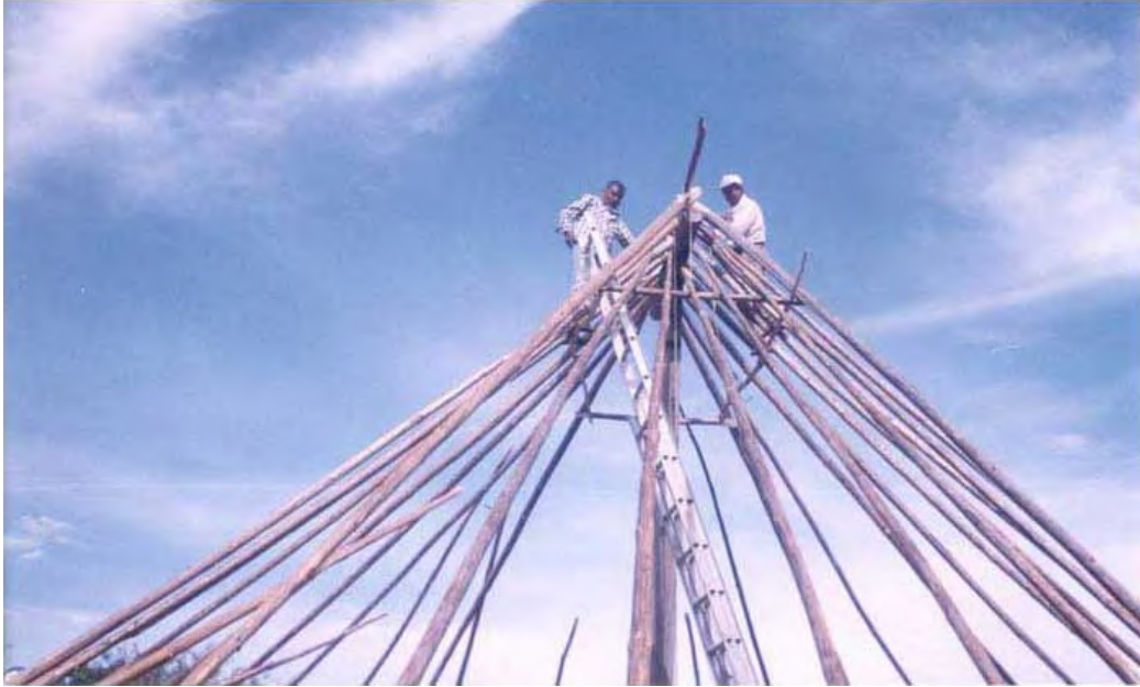
Figure 30. Temple's roof structure. Photo provided by Mr. Pablo Muñoz.
