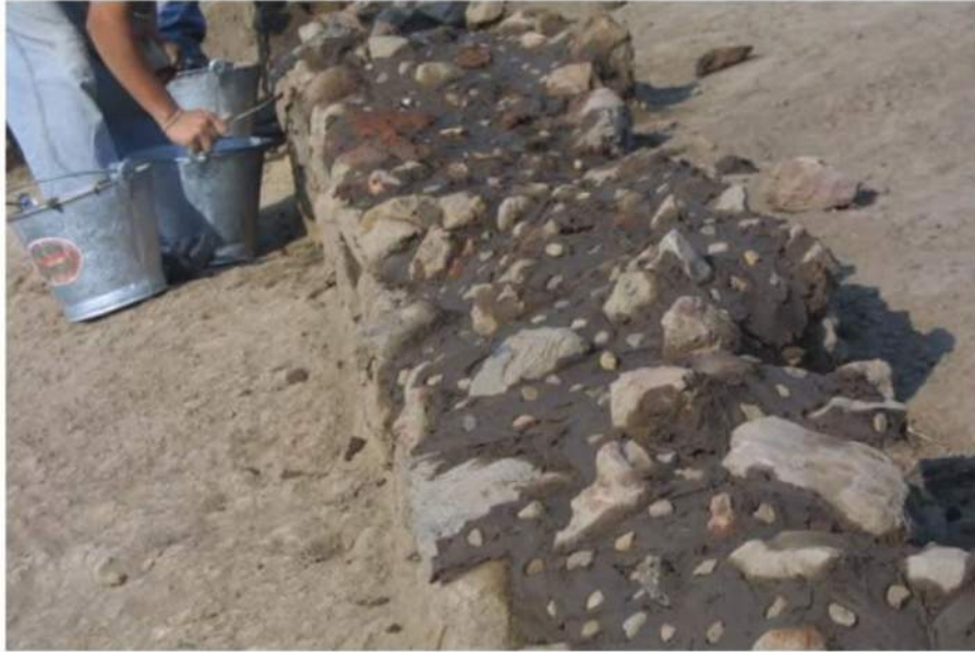
Photo 23. Consolidation of the walls.
