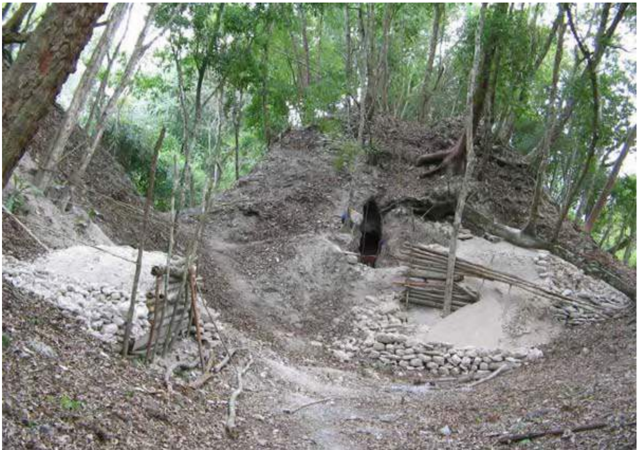
Figure 48. Looting in building B-16.
