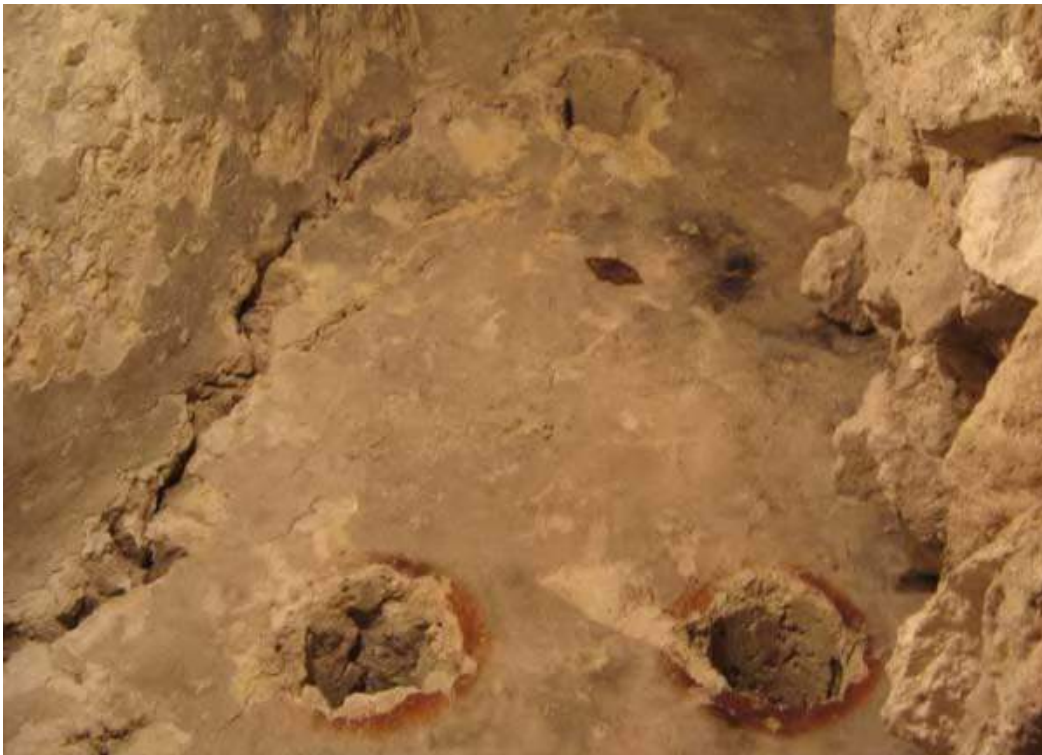
Figure 32c. Palace B-15: vault of north precinct, second level.
