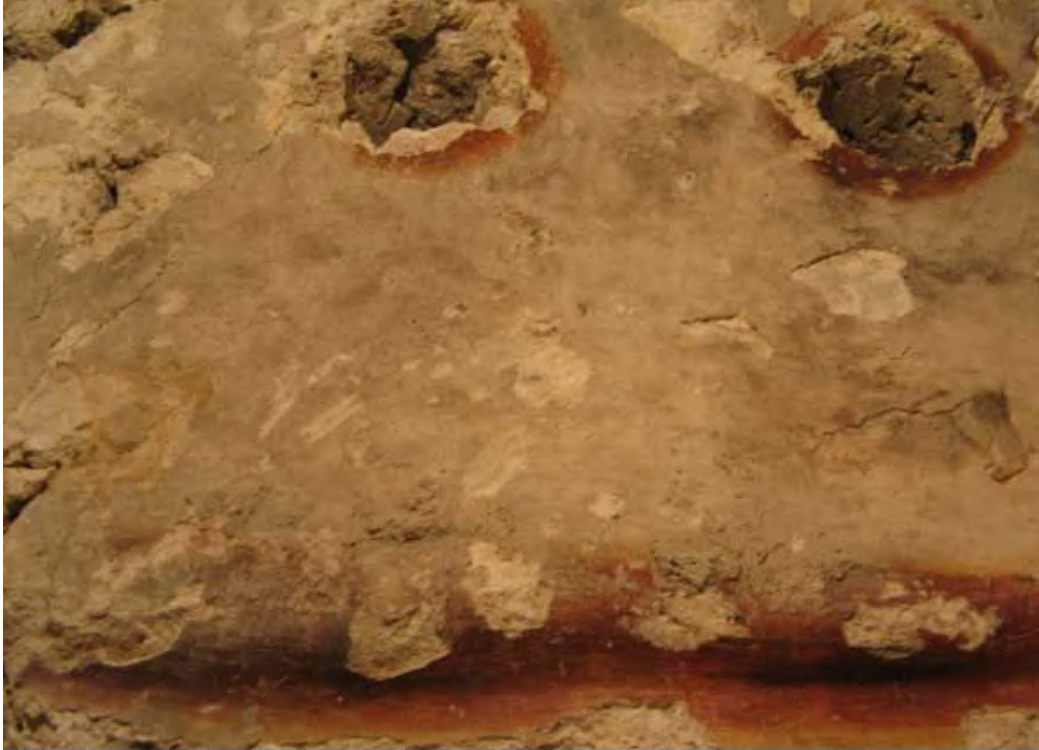
Figure 32b. Palace B-15: vault, soffit and holes for rafters.
