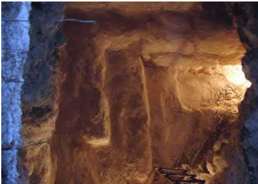
Figure 37. Structure B-sub 1, tunnel (view toward east).
