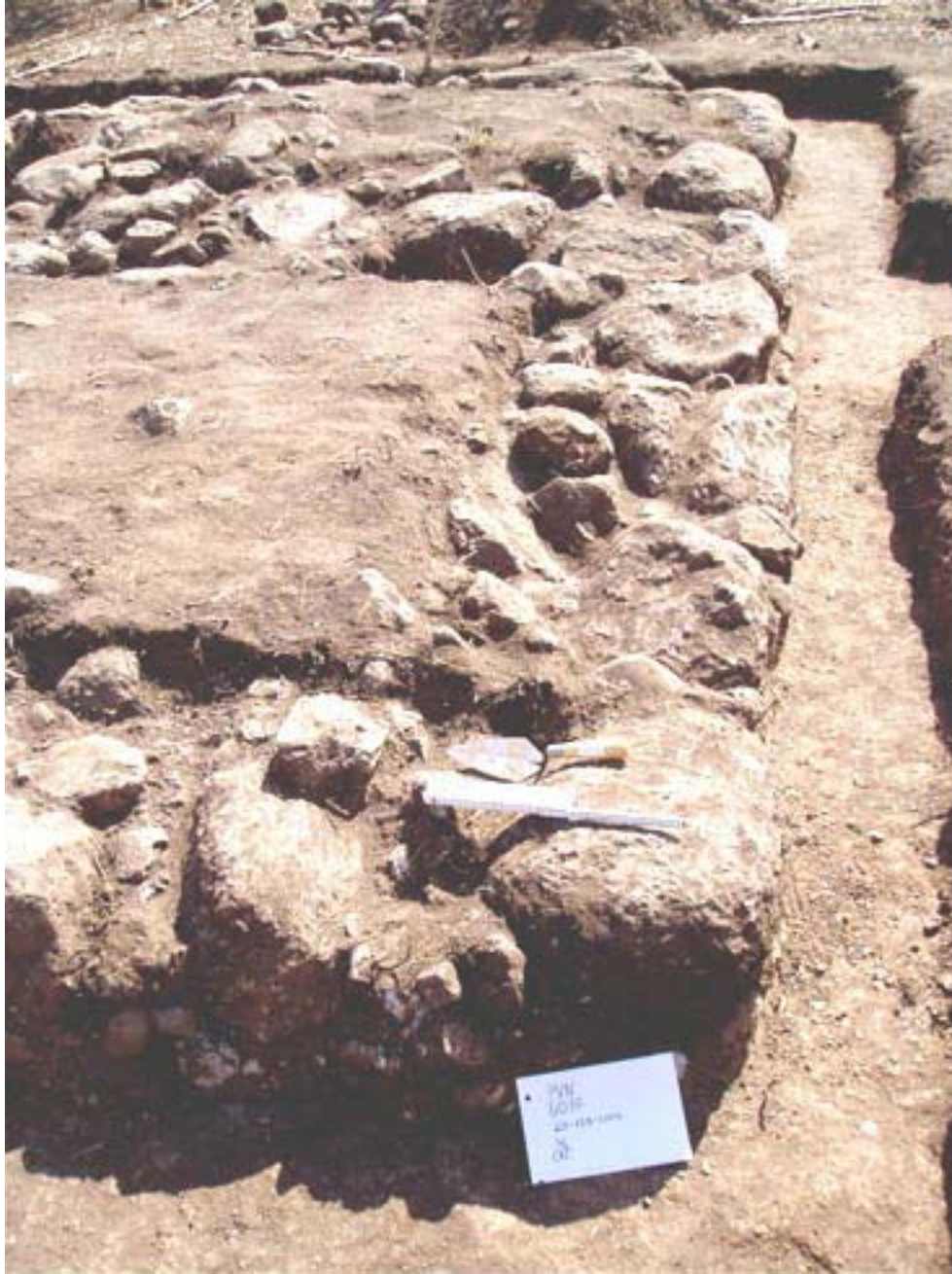
Figure 8b. Site PVN 607, Str. 3, Detail, West basal wall, northwest corner in foreground.
