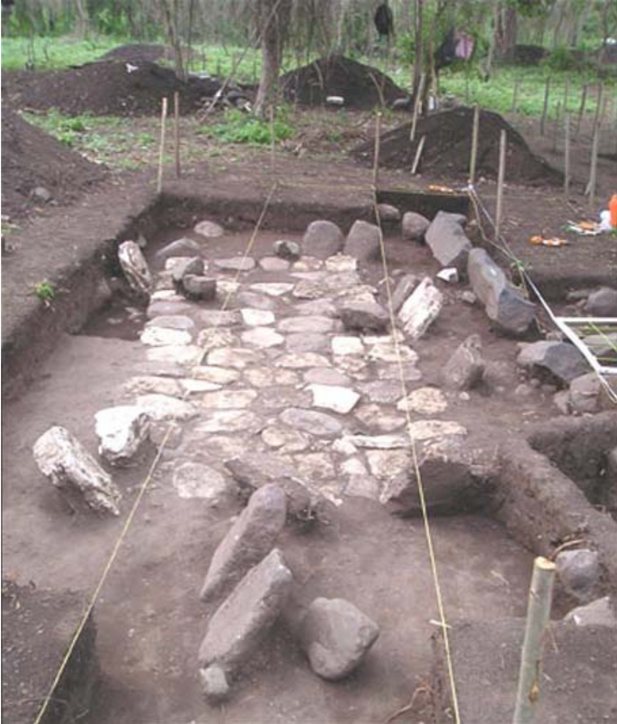
Figure 45b. El Coyote, Pavement in copper processing area: Close-up, pavement, showing use of vertical edging stones and placement of columnar basalt.
