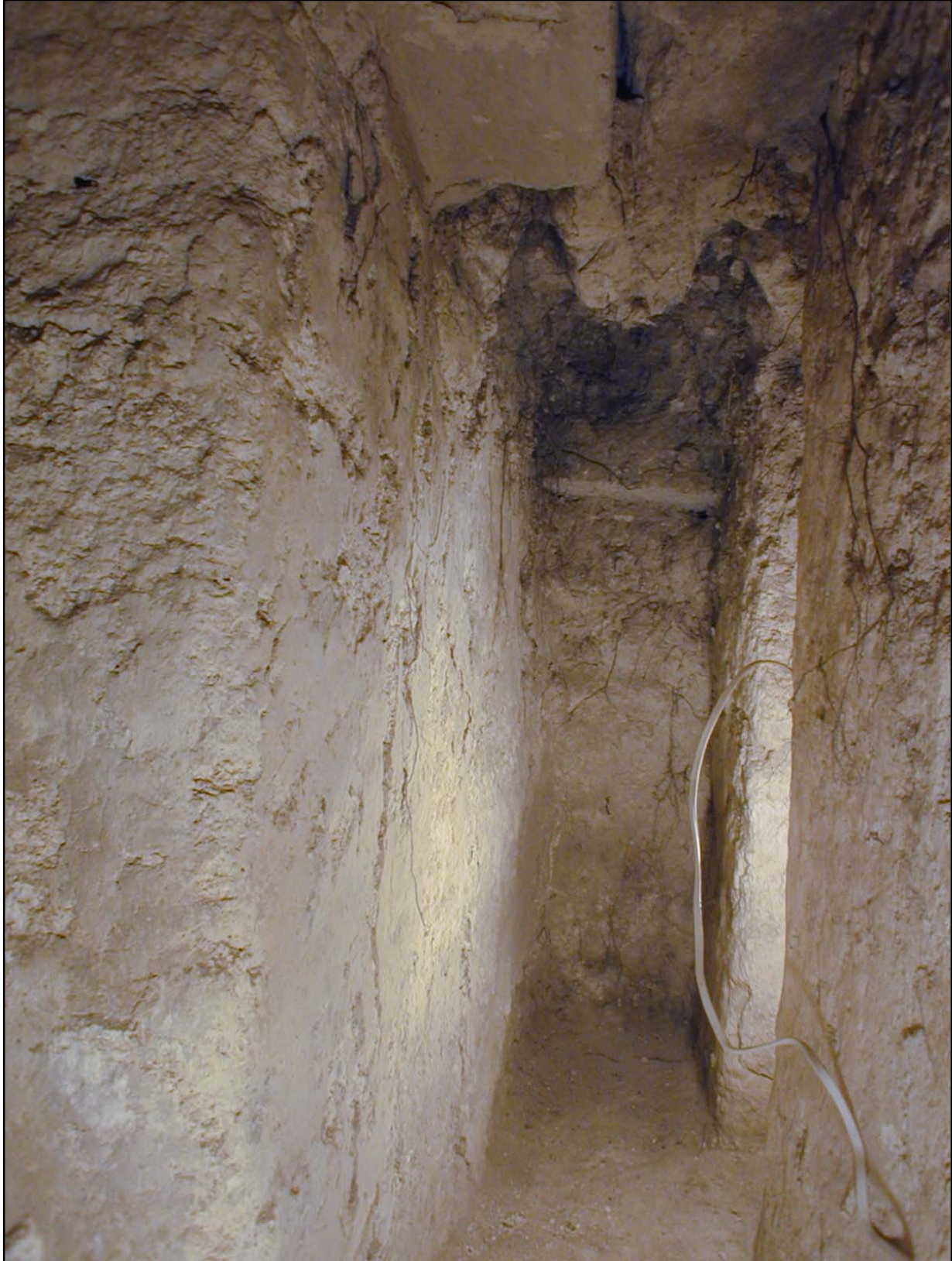
Figure 12 Eastern wall of Structure 1 sub 3 with doorway leading to Structure 1 room 3 to the east
