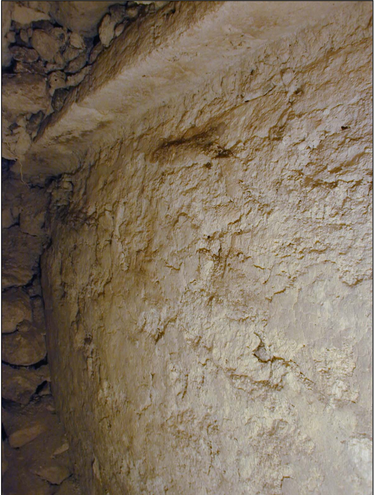
Figure 13 Southern wall of Structure 1 sub 3 with cornice
