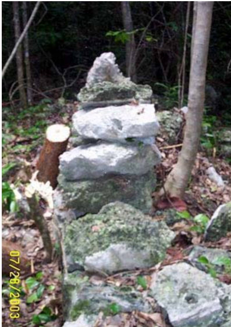
Figure 8. Simple stone wall (albarrada) formed by a single line of dry-laid boulders.
