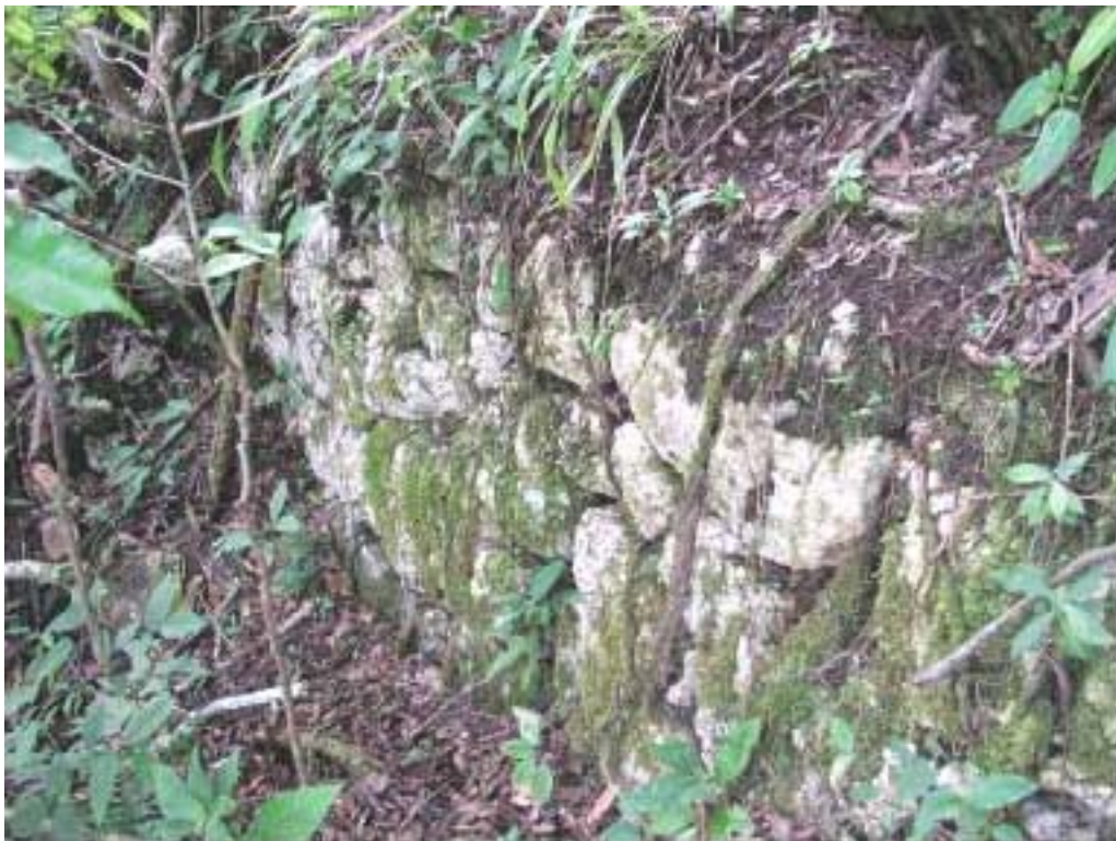
Plate 26. Álvaro Obregón 2 platform wall.
